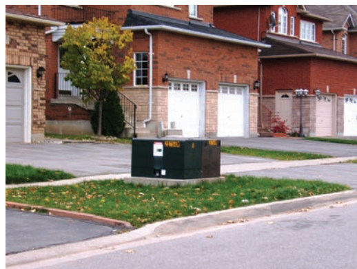
Pad mounted transformer
