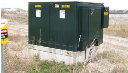
Pad mounted switchgear
