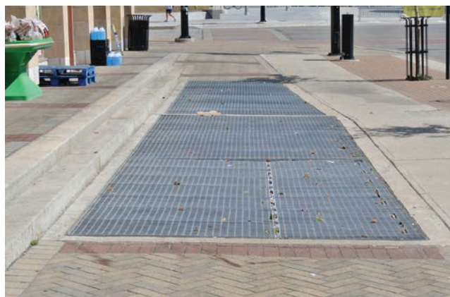
Sidewalk grates used for transformer access and ventilation
